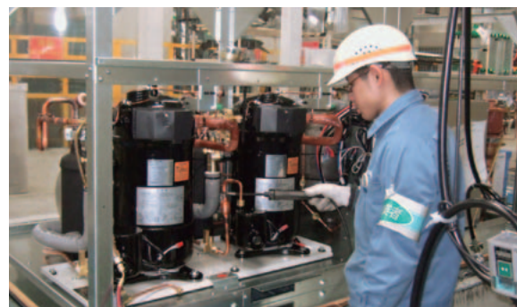
Refrigerant leak inspection process using helium gas
